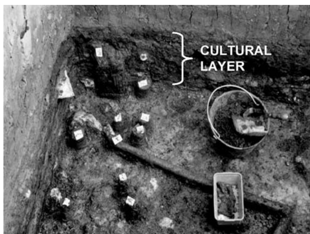
Fig. 5 Wooden piles in the excavation trench from Hočevarica, recovered within the cultural layer. They mostly belong to Fraxinus ornus/excelsior and Quercus robur/petraea (after Čufar and Velušček 2004)
